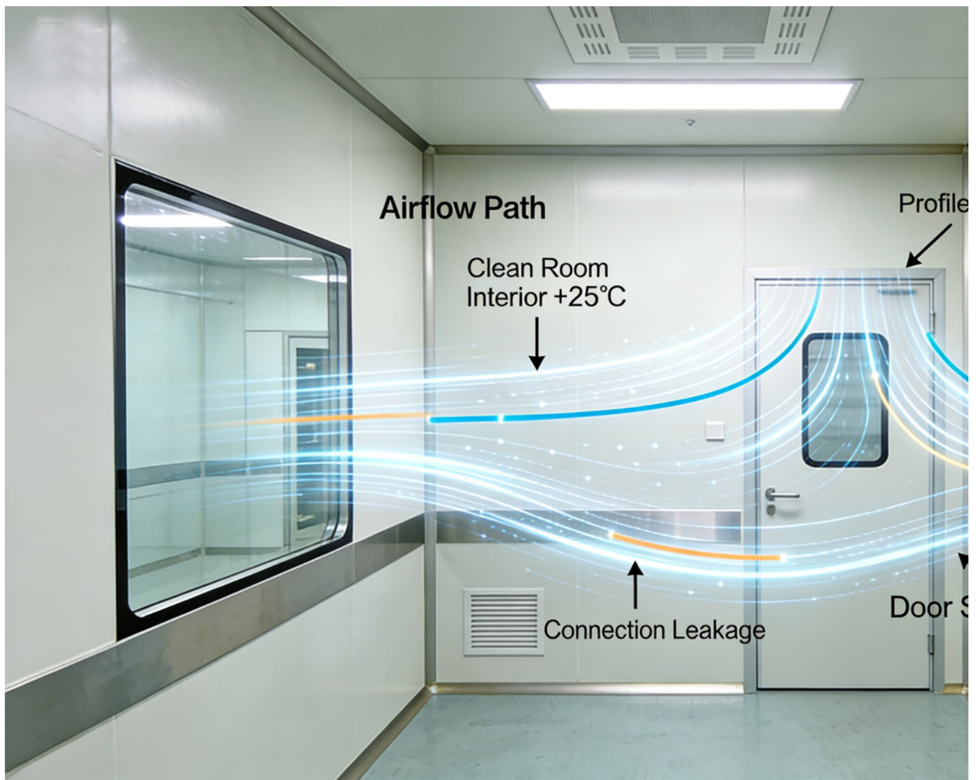
Figure: Air leakage paths in a pressurized CleanRoom
